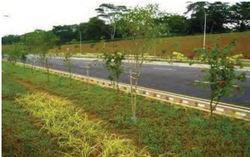
Bioretention swales @ Sengkang West Way
